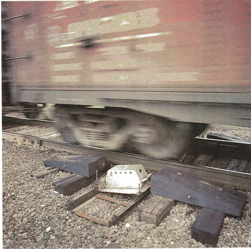
Hotbox detector on the Santa Fe. New trackside devices now in use or under test monitor other types of mechanical failures that can cause costly accidents.
